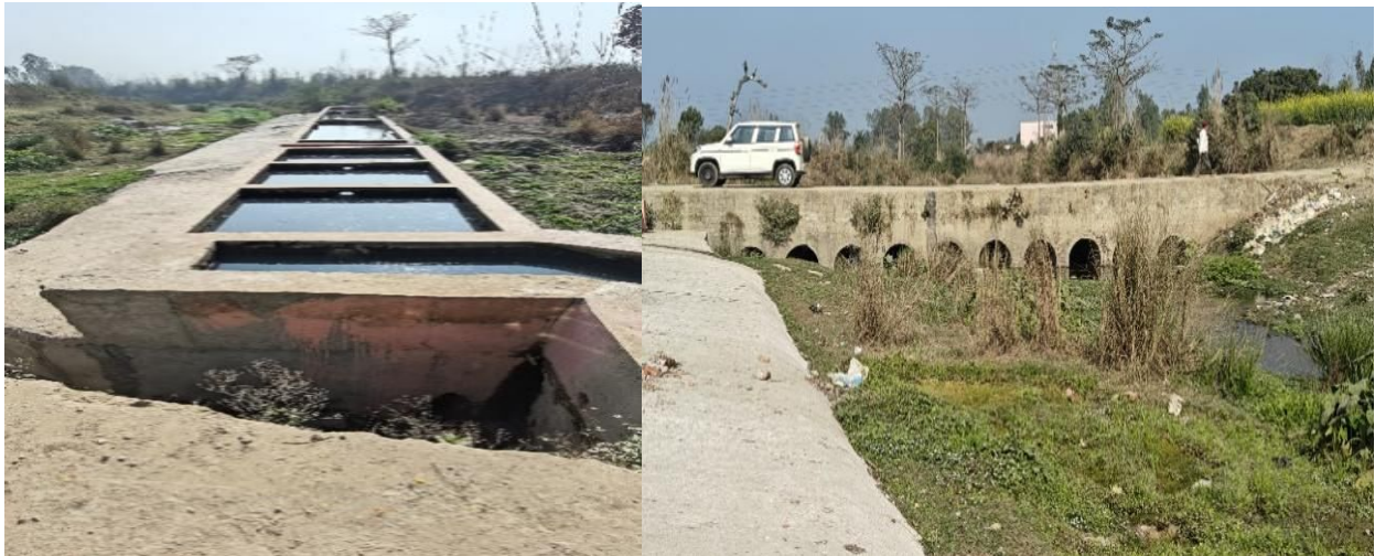
Constructed wetland situated in Madh village
